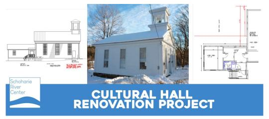
The SRC Cultural Hall was built in 1857 by local carpenter Boss Jones and is a classic federal style timber frame construction building with King Post Trusses. Planned renovations include:
